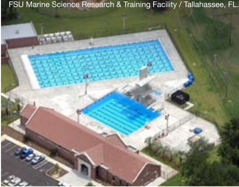
FSU Marine Science Research & Training Facility / Tallahassee, FL.
